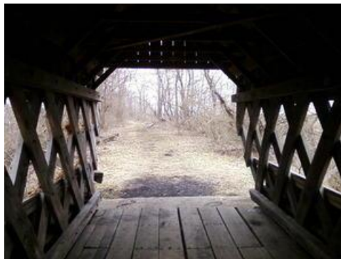
Covered bridge at The Ohio Canal Greenway on the Hebron Trail
