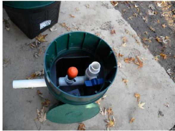
**Figure 8. Turn-up and 3/4 inch air gap/ bleeder at the end of each lateral for routine maintenance**
