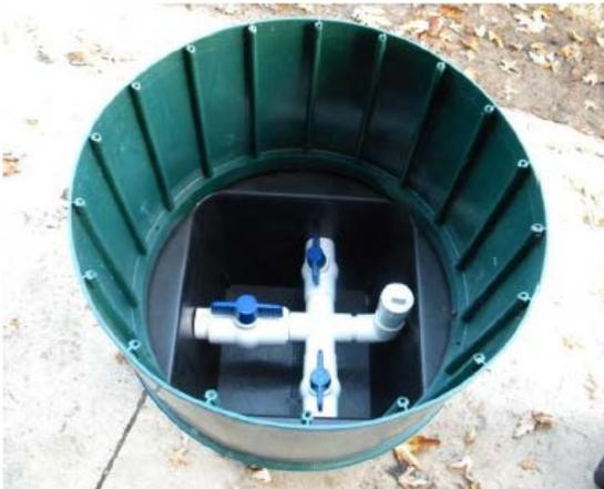
**Figure 7. Service box within the manifold line.**
