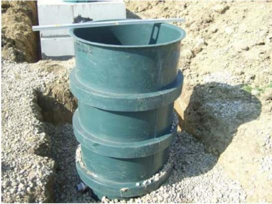
**Figure 5. Dosing siphon - external view**
