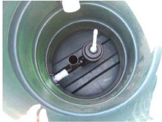
**Figure 6. Dosing siphon - internal view**
